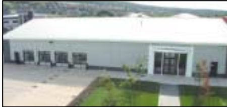
Left: AESSEAL® API682 Version 2 Test Facilities
